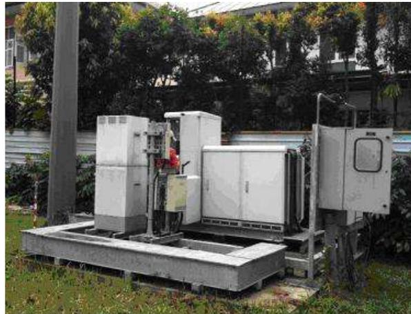
**Figure 8: Electrical facility, SMR often suffer lightning surge interference**
