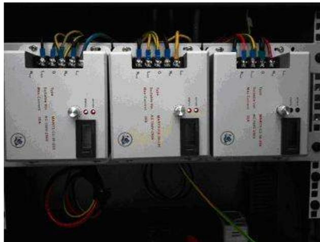
**Figure 9: 3 sets of SET with surge counter were installed in SMR of Figure 8.**
